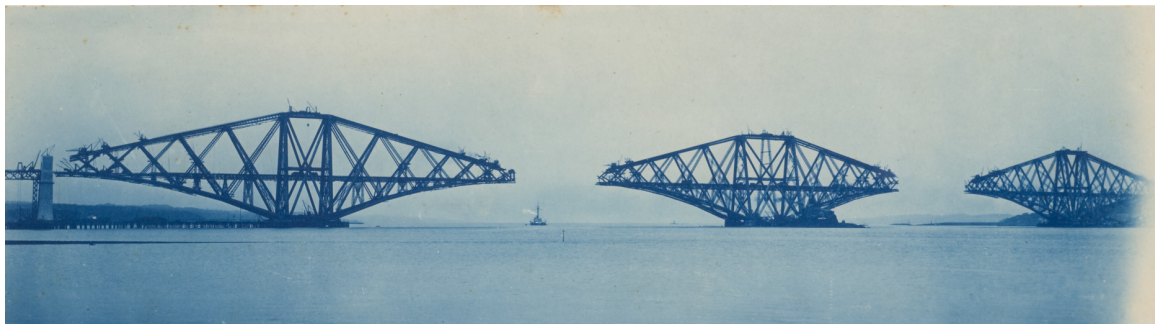
Fig. 5.13 Evelyn George Carey, Construction of the Forth Bridge (Collection of the Canadian Centre for Architecture)
